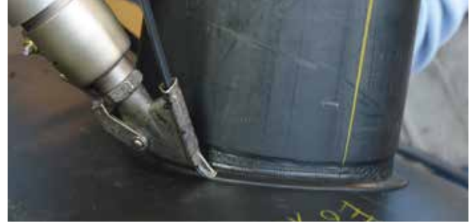
Draw welding with combination nozzle.
