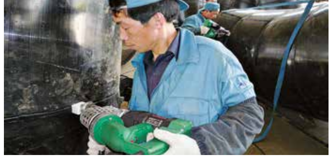
In operation during container construction in China.
