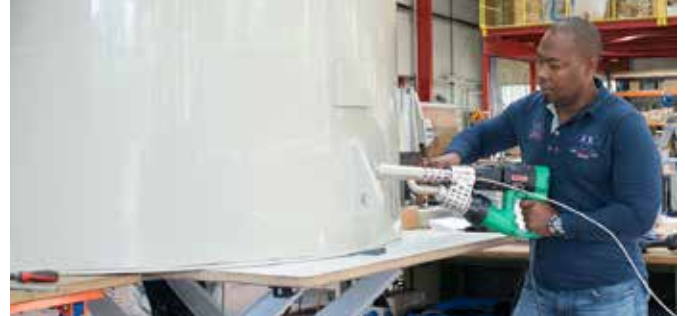
FUSION 3C during the welding of a fillet weld.
