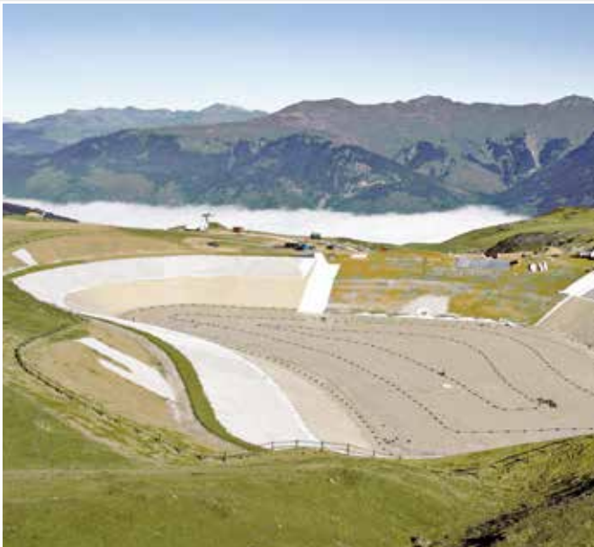
Water Reservoir HDPE 2.0 mm
