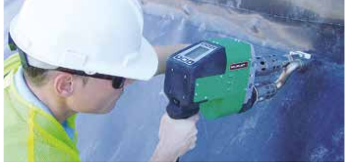
The powerful WELDPLAST S4 at work.
