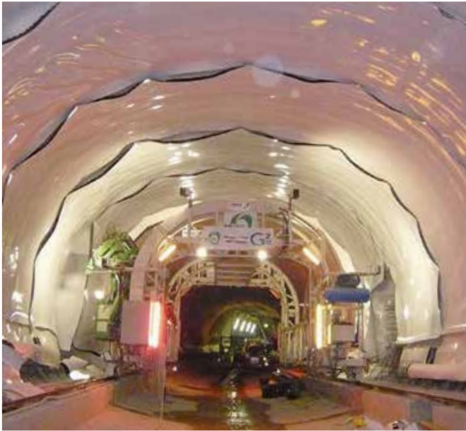
Tunnel PVC 2.5 mm
