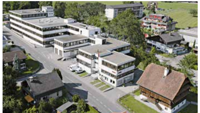
Leister Technologies AG, factory, Kaegiswil, Switzerland
