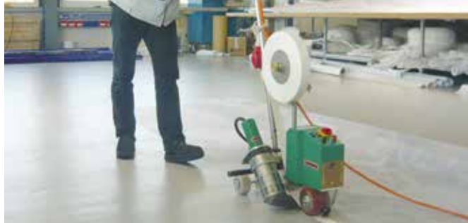
Welding tape at maximum speed.
